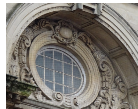
Local built character
