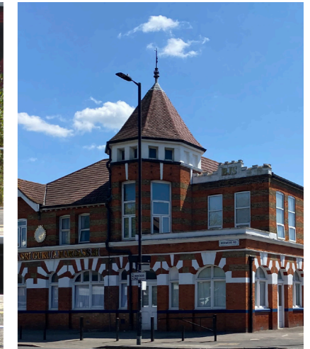
Local built character
